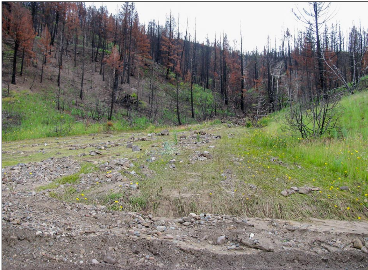
FIGURE 14 Deposition zone of a post-wildfire debris flow onto Dog Creek Road (berm of road in foreground), following the 2010 Place Lake Fire. (Photo: B. Chapman)
