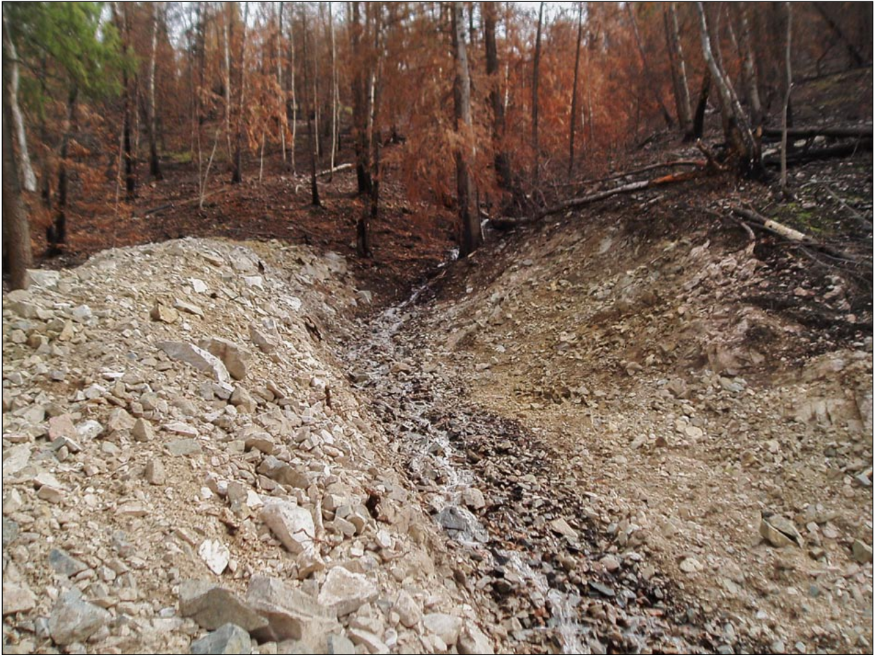
FIGURE 11 Debris flow deflection berm constructed to protect a residence at risk below the 2009 Terrace Mountain Fire. (Photo: T. Smith, Westrek)
